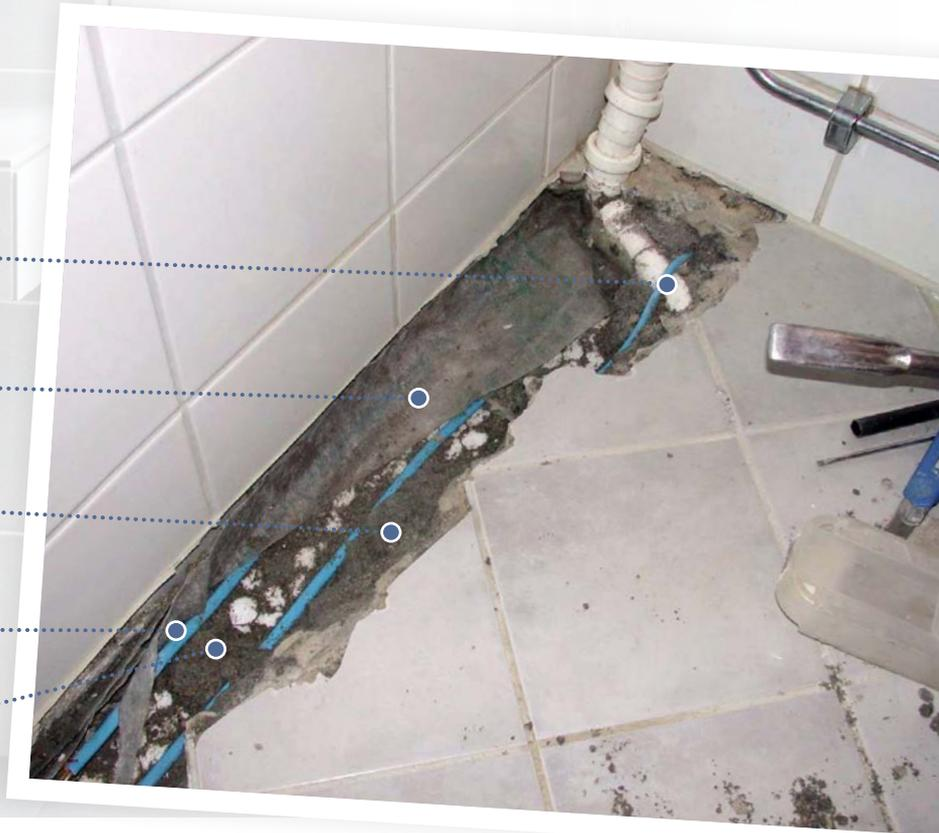
Cable in direct contact with thermal barrier (PVC-pipe)
