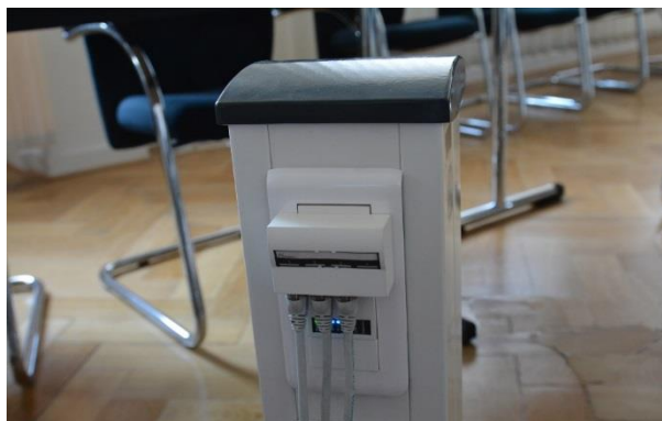
Figure 9: Communication pillar installation
