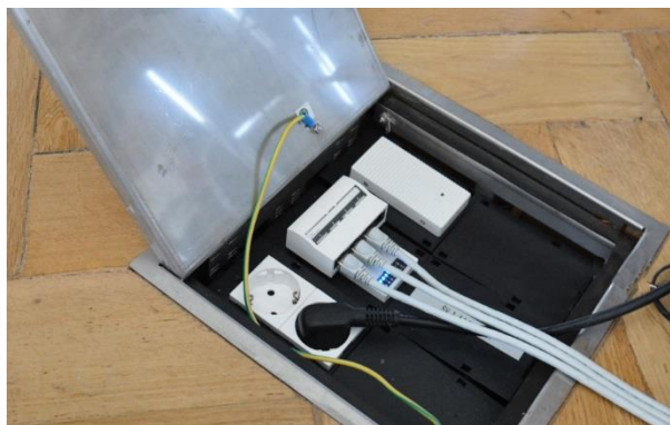
Figure 5: Floor box installation
